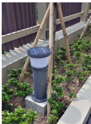
Solar powered LED bollard light
